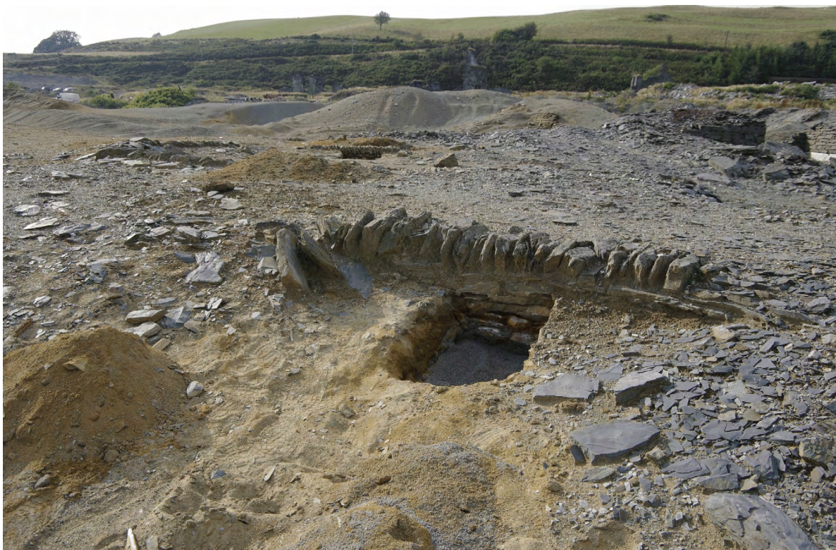
No. 1 [above, to N]: complete stone outer wall, no remains of wooden deck. No. 2 [below]: only a small part of the outer wall at the northern end remained.
